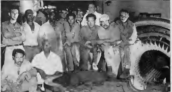
Shown above is a 75,000-kilowatt generating unit at No. 2 Powerhouse which is open for inspection by a group of employees under the direction of Ernest Ball, International General Electric representative. To the right is the armature of the generator, and in the foreground is part of the steam turbine. Mr. Ball will spend six or seven months in Aruba inspecting the various GE units in the refinery. In the group above are C. Jacob and C. Hughes, kneeling; standing from the left are A. Casali, I. Warren, R. Milas, H. Nixon, E. Maduro, R. Vanderlinden, Mr. Ball (behind Mr. Vanderlinden), G. Holman, and A. Briesen.
